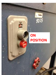
Figure 5. Equipment in ON position. Black START button compressed.
